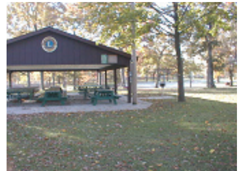
Pavilion at Goold Park
