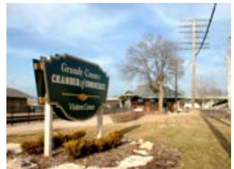
Existing Morris Railroad Station
