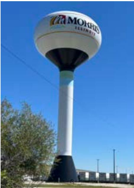
New Water Tower Near the Costco Warehouse Campus
