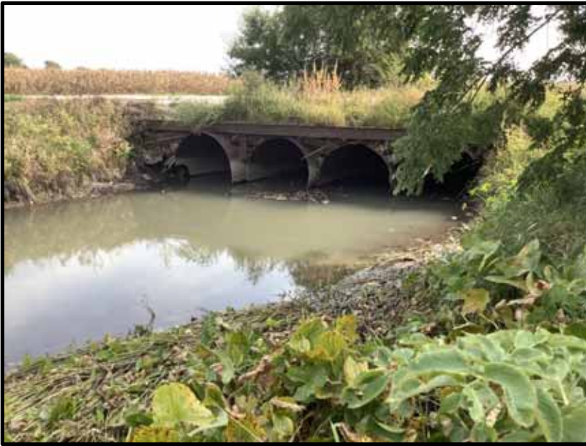
9. View downstream of Valley Run towards Ashley Road.
