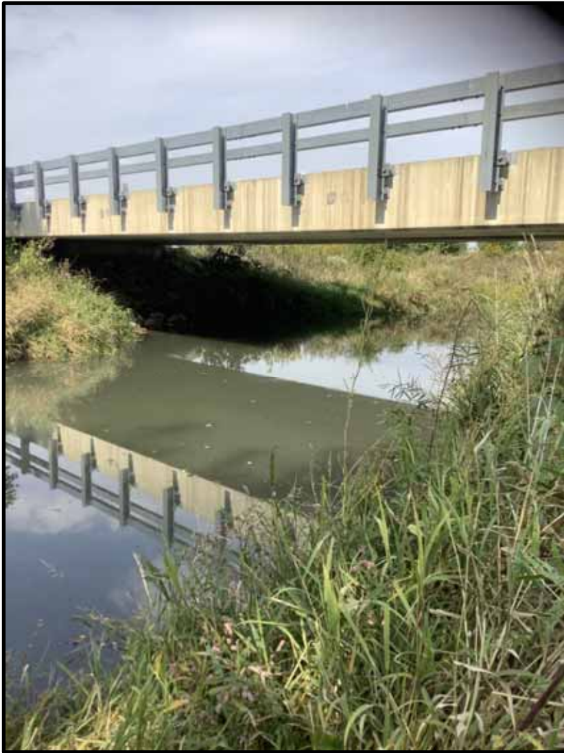
5. View upstream of Valley Run toward Whitman Road bridge.
