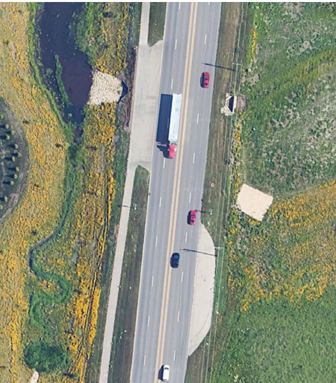
Figure 18. Truck Pullouts in Kane County, IL
